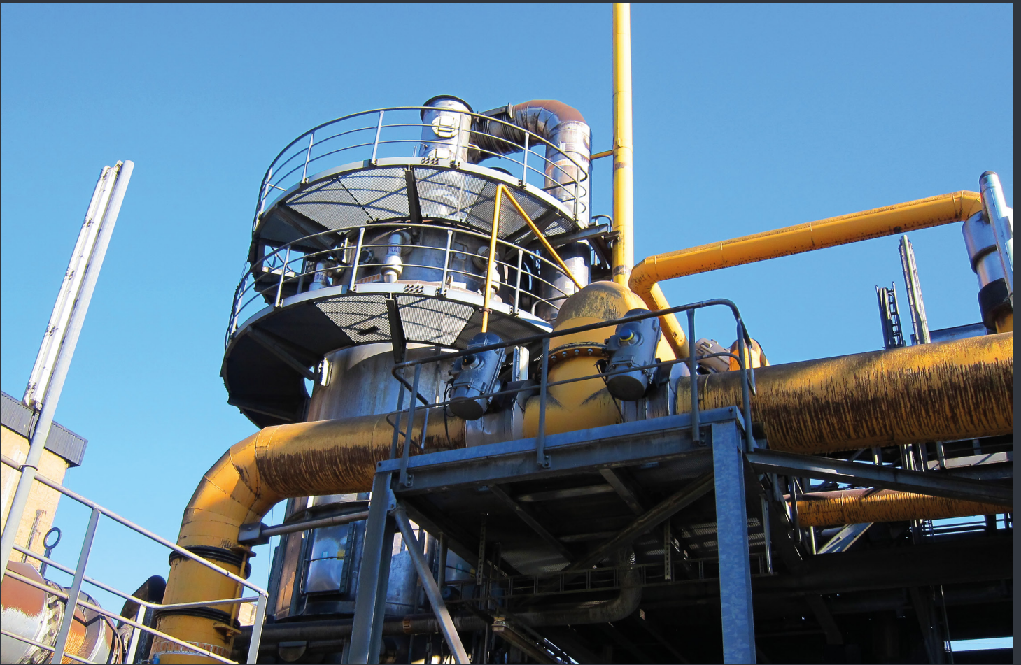
Daily flushing of the electrostatic filter with hot water has been a success.
