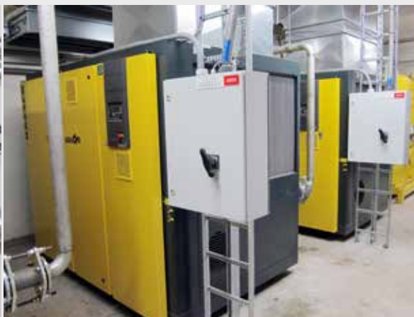
The new "Heating Central" that will receive and heat-exchange the hot cooling-water destined to both the hot-water tanks and to the ventilation system in our wardrobe building
